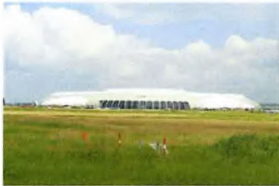
Sprung Instant Structures in the Highway 2A Corridor
