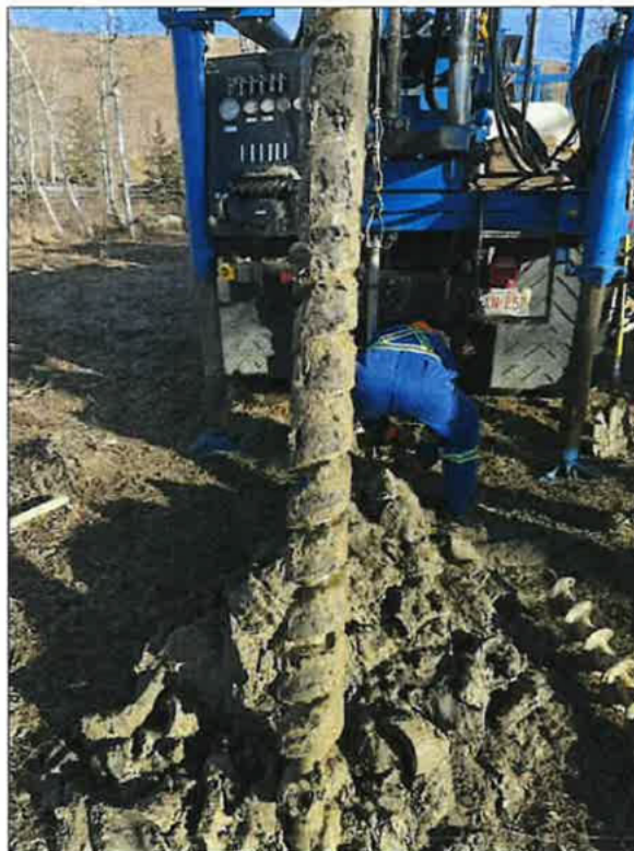
FEB. 11, 2026 - BH01 RETRIEVED SOIL SAMPLES.
