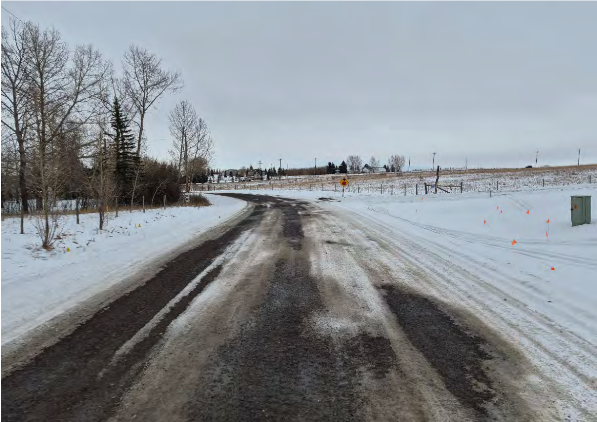
Figure 3 - Site Photo – Looking East - Approaching 32 nd Street East
