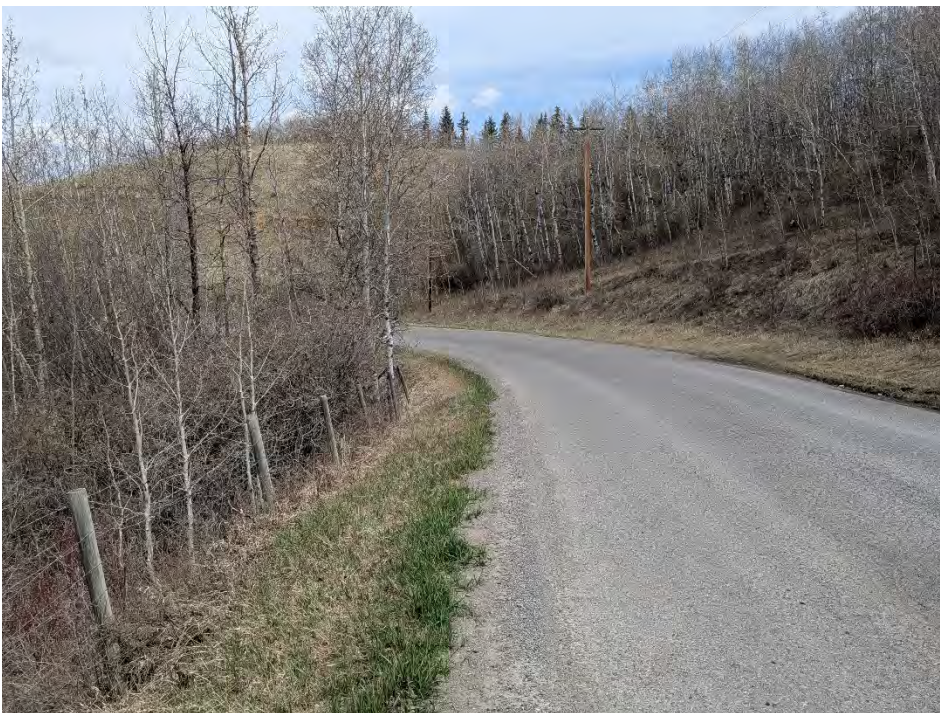
Figure 5 - Site Photo – Looking Northwest
