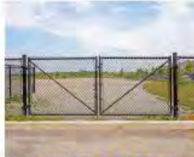
6 foot tall double swing gate at the entrance of each dog park and buffer zone.
