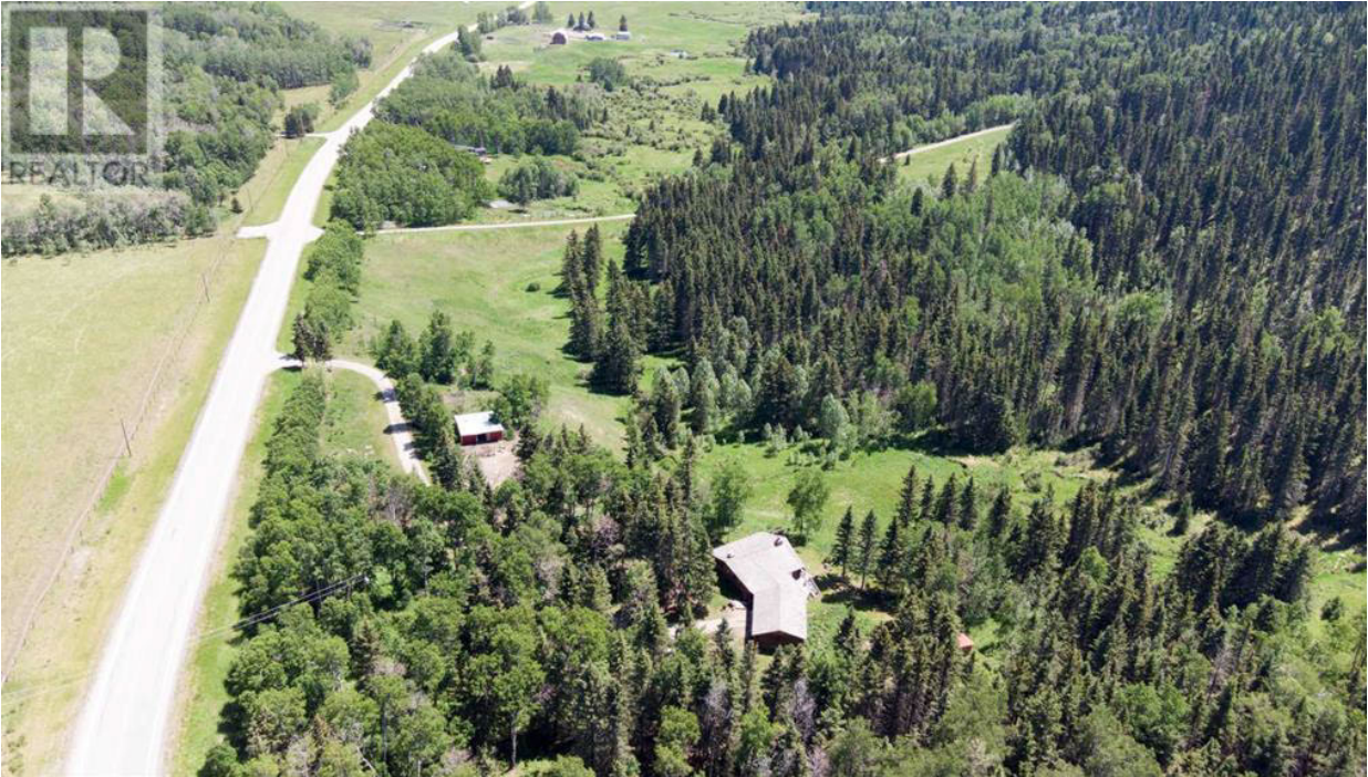
Photo 1: Existing Yard Facing East
