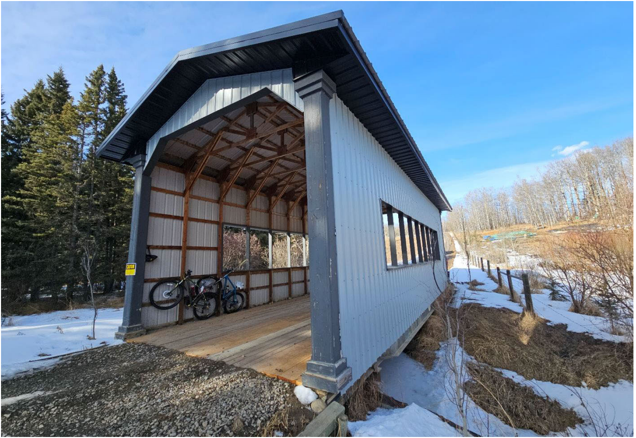
Photo 17: SE Corner of Bridge
