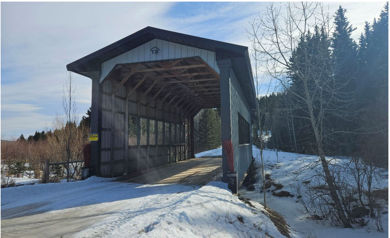
Photo 16: North Face of Bridge
