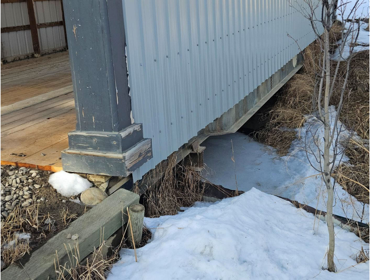
Photo 19: Bridge "I" Beam on Steel Piles
