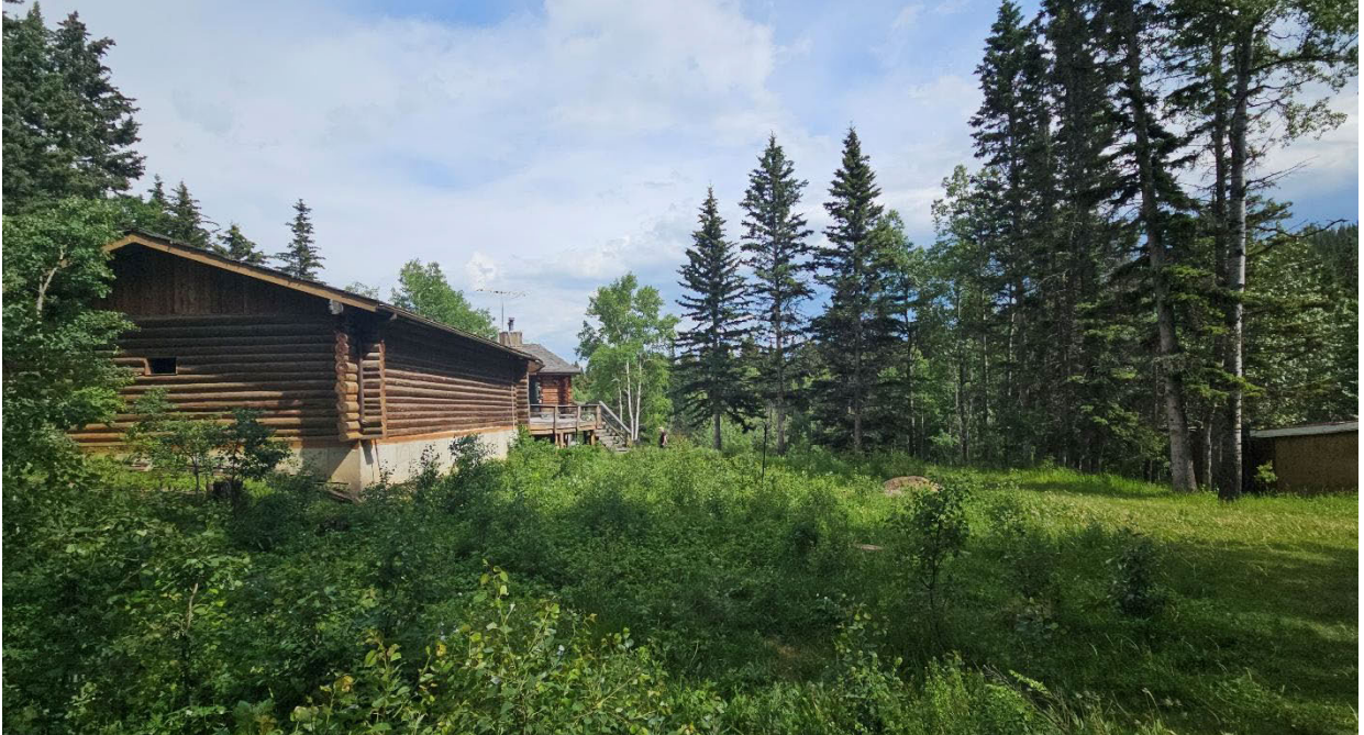
Photo 9: House Facing East
