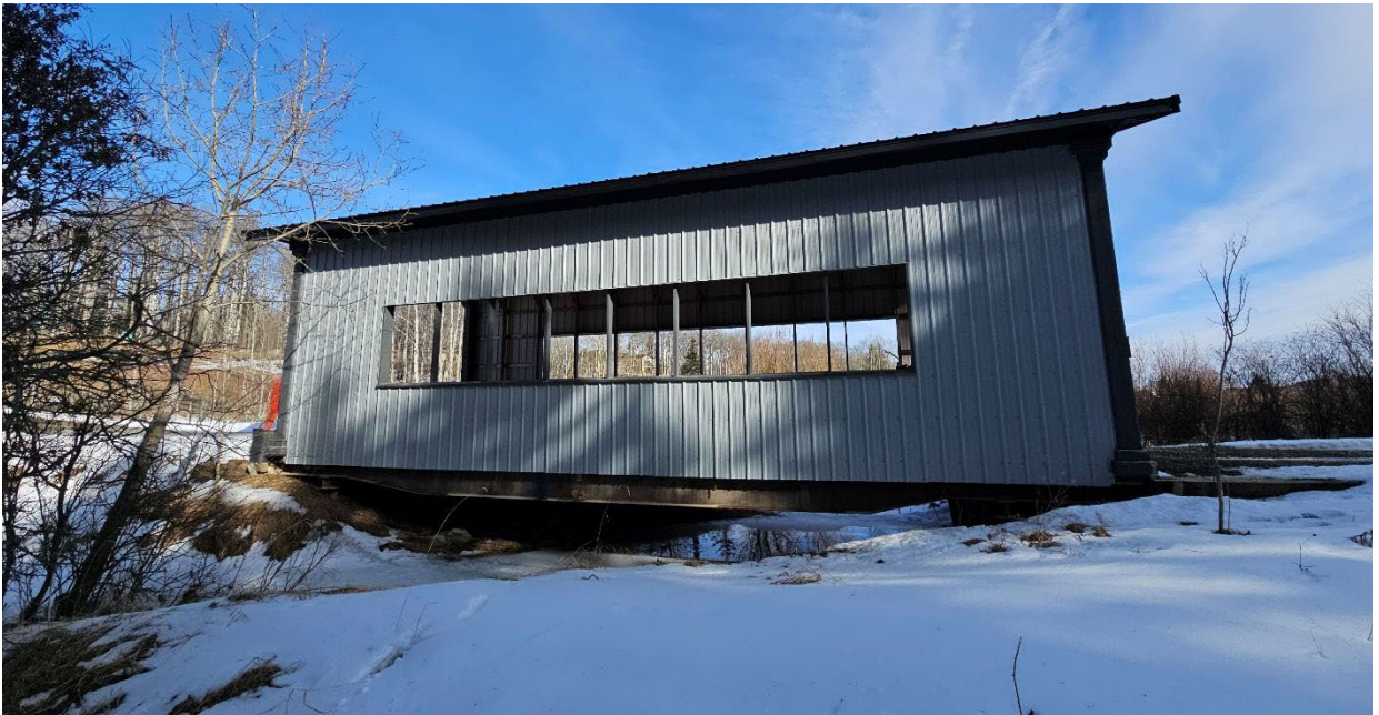
Photo 18: West Side of Bridge
