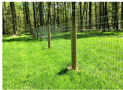
4 foot no climb mesh for the perimeter fence
