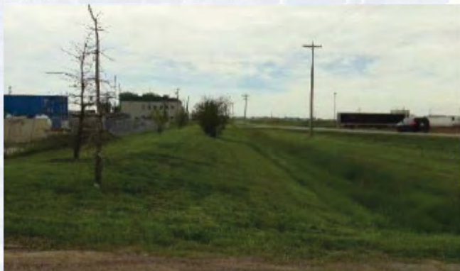
Roadside ditching for stormwater conveyance
