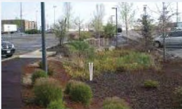
Vegetated drainage swale
