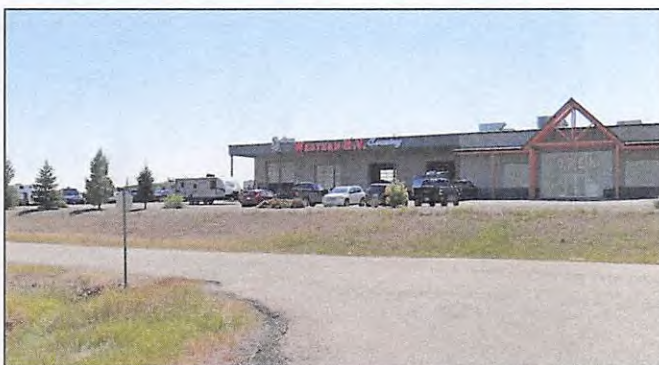
RV SALES & STORAGE PORTION OF SUBJECT SITE
