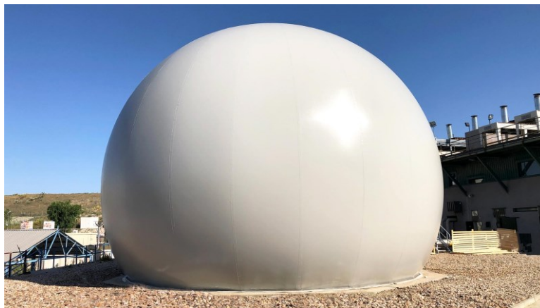
Figure 13: biogas gasholder with 2-layered membrane
