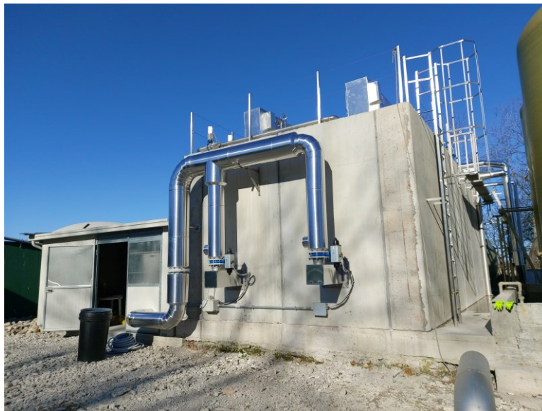
Figure 11: An Ammonia stripping system to pull out excess nitrate
