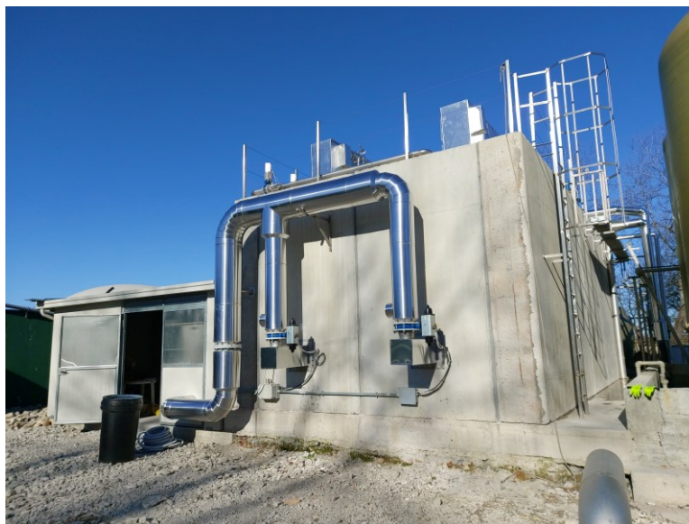
Figure 11: An Ammonia stripping system to pull out excess nitrate
