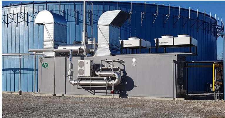
Figure 18: Cogeneration System supplies both thermal and electrical energy
