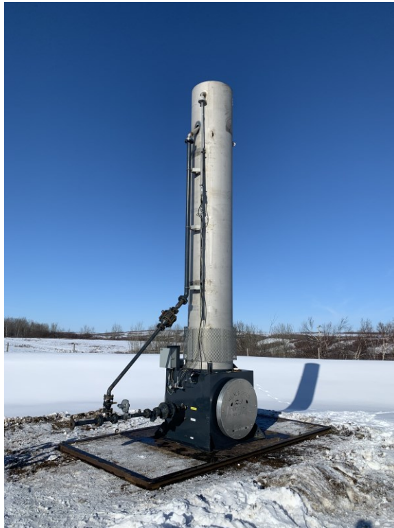
Figure 17: Example of a safety flare
