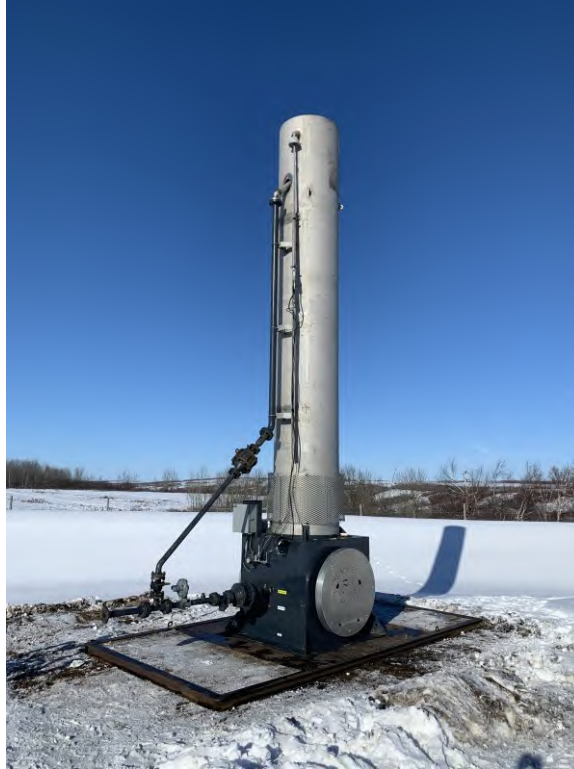
Figure 17: Example of a safety flare
