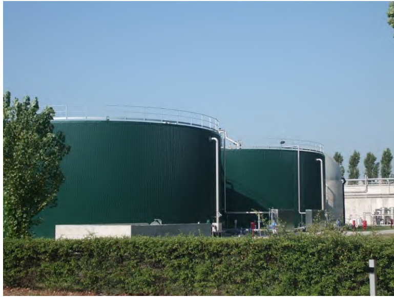
Figure 7: Example of anaerobic digesters and associated heat exchangers
