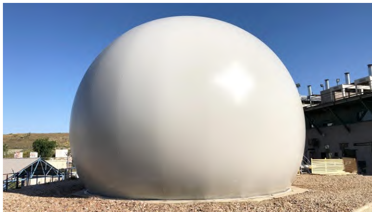
Figure 13: biogas gasholder with 2-layered membrane
