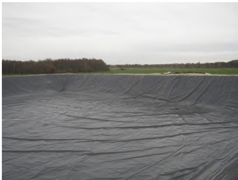
Figure 12: Empty Lagoon with liner
