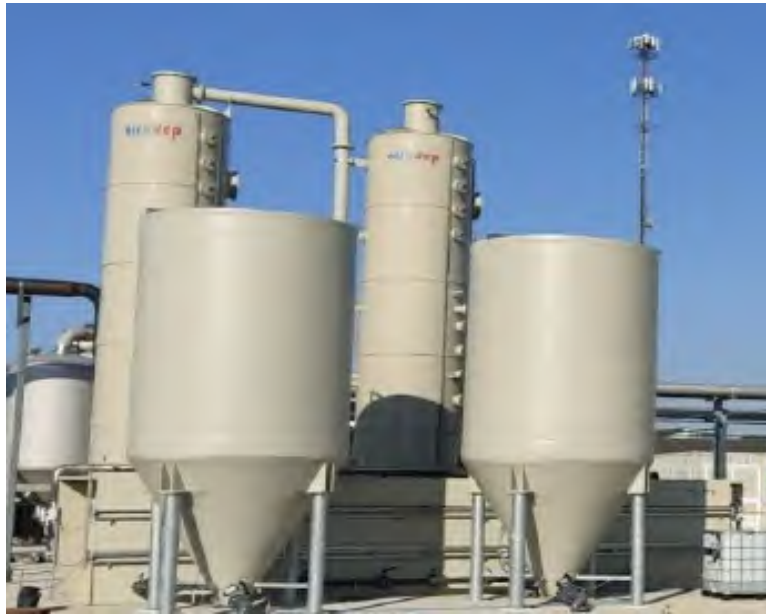
Figure 14: A two-stage H 2 S scrubbing system
