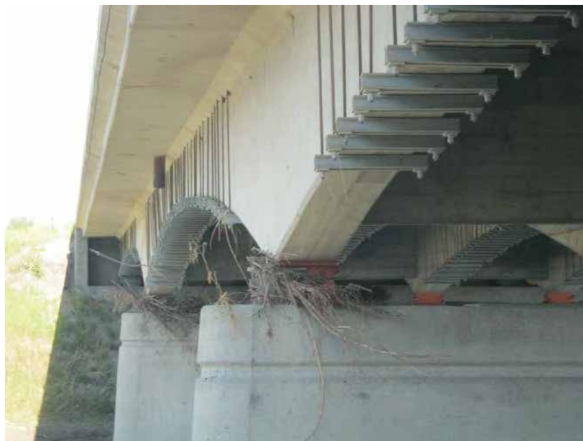
Photo 11 Looking west along south side- HWM drift on pier seat- 300mm high.
