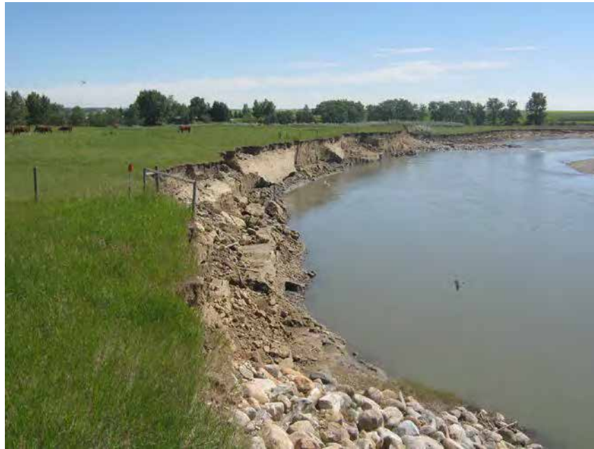
Photo 9 Scour at n.w. bank looking north from bridge.
