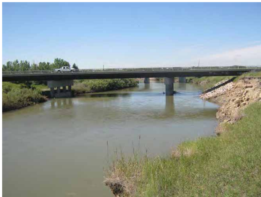
Photo 7 Looking u/s at bridge from n.w. bank- scour at n.w. bank.
