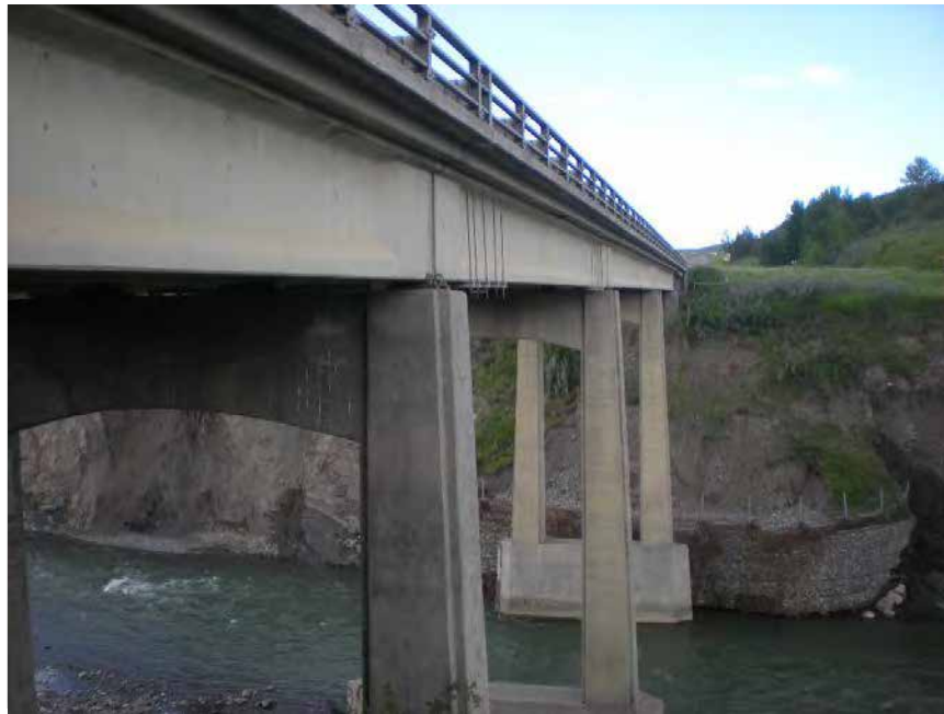
Photo 3: From SE abut. embankment looking north at east d/s girder line. Horizontal and vertical alignments are good. Gabions in place at north headslope but may be missing riprap at U/S end.
