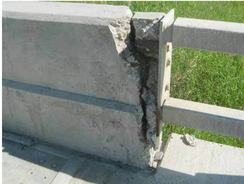
Photo 9 Parapet broken at n.w.
