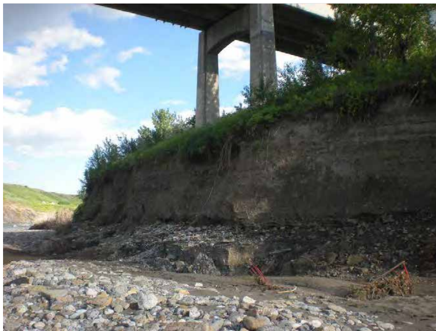
Photo 6 Looking d/s from SW bank at erosion at south headslope - beneath P1.
