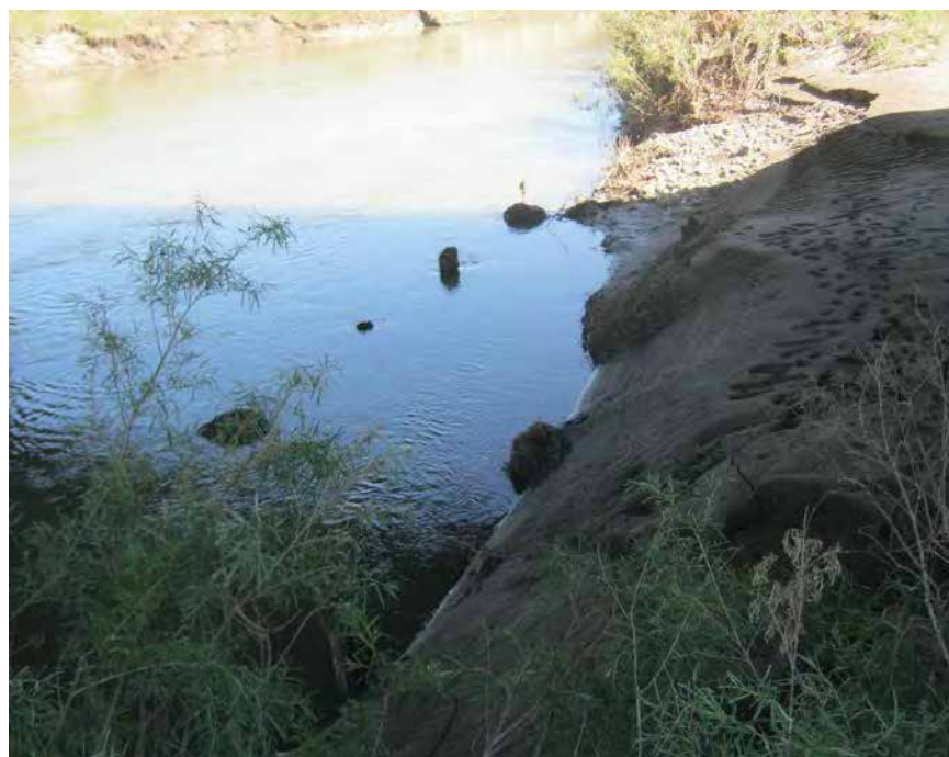
Photo 12 Minor scour at east bank under bridge.
