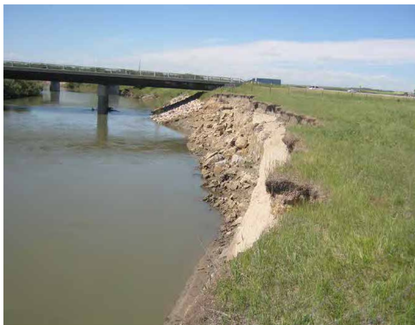
Photo 8 Scour at n.w. bank looking south towards bridge.
