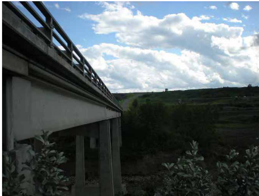
Photo 1 From NW abut. embankment looking south at west girder line. Horizontal and vertical alignments are good.
