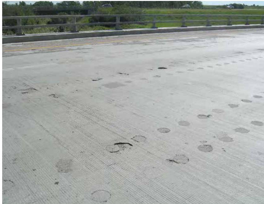
Photo 8 Patched core hole spalls in deck.
