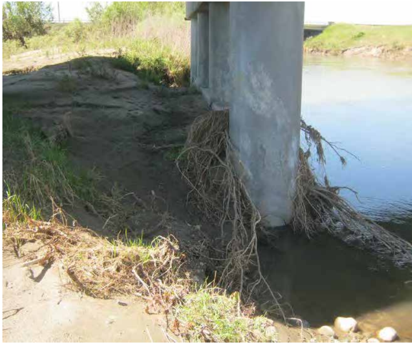
Photo 11 Localized scour at ends of P2.
