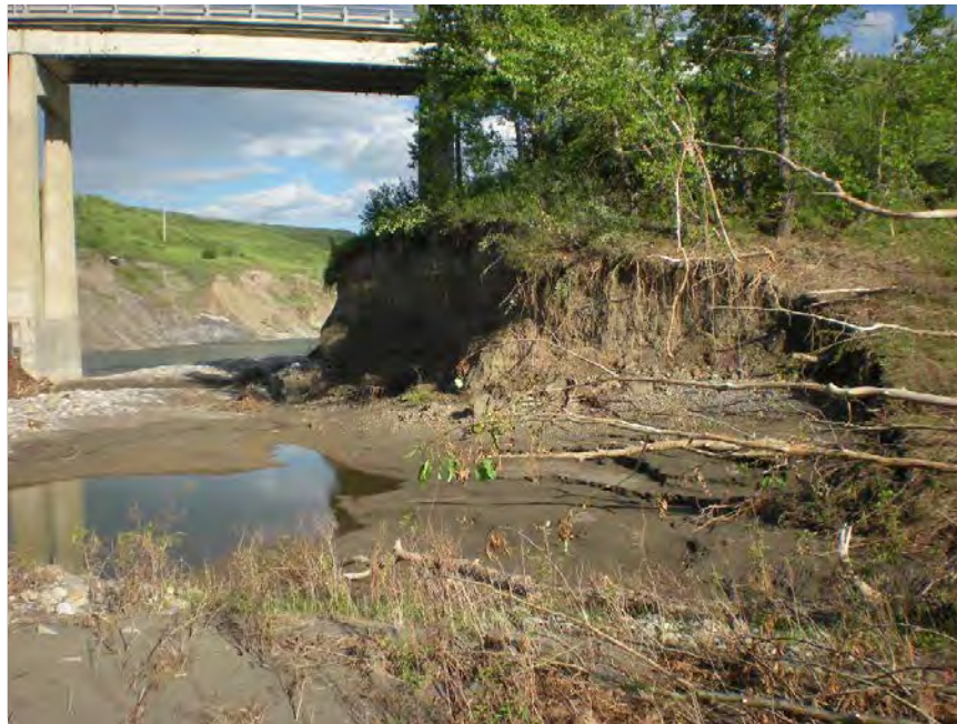
Photo 7 Looking d/s from SW bank at extent of erosion around SW corner.
