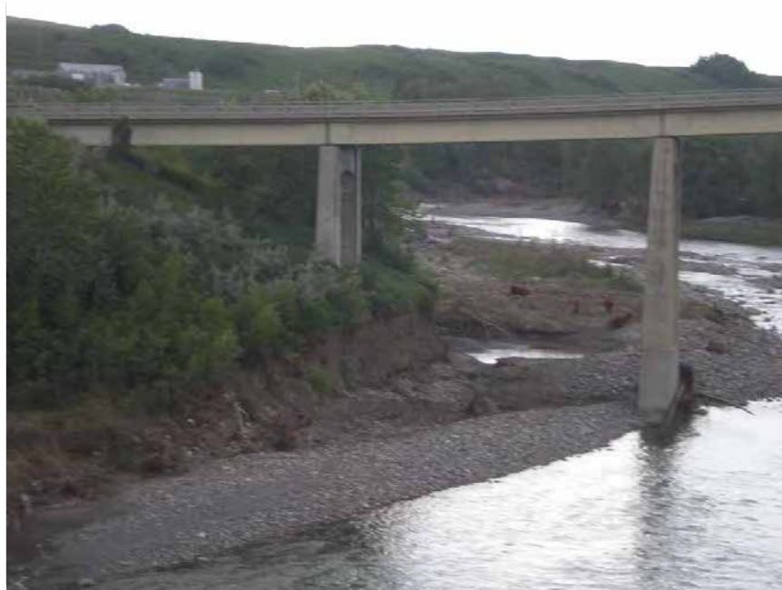
Photo 5 Looking u/s from NE bank at P1 and P2, note erosion under P1.
