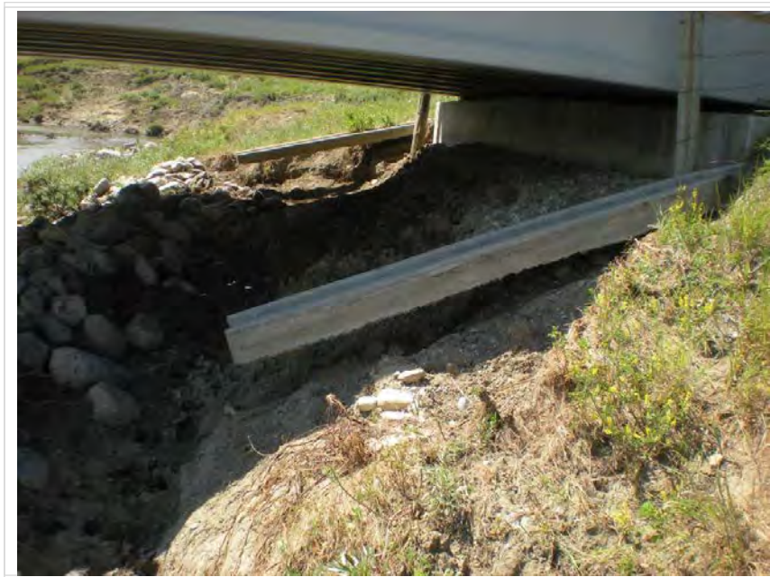
Photo 5 North headslope erosion and hanging drain troughs - replacement fill and scour protection required.
