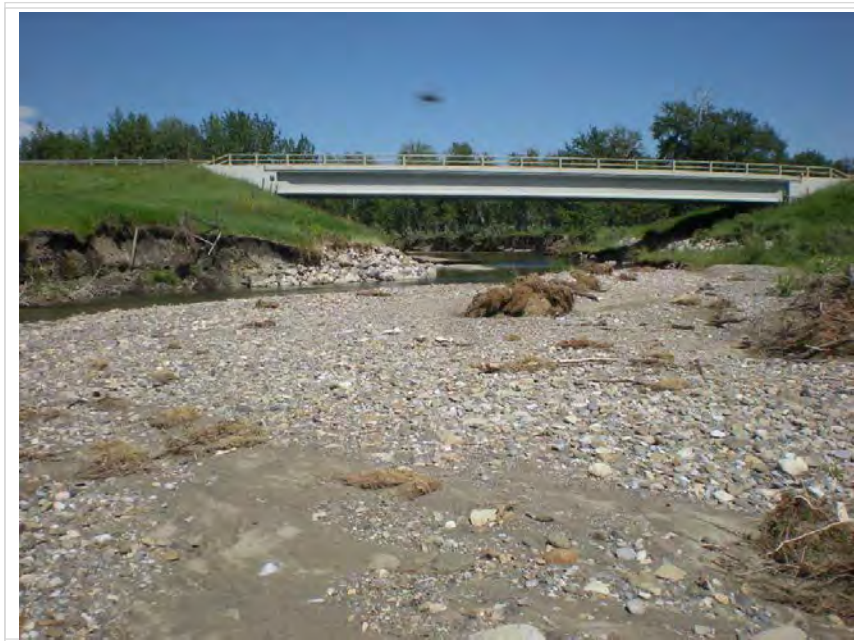
Photo 5 Scour at NW embankment 30m upstream of bridge.
