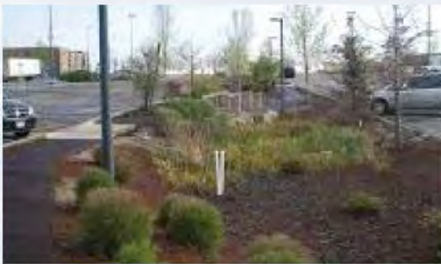
Vegetated drainage swale
