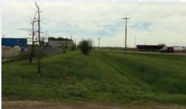
Roadside ditching for stormwater conveyance
