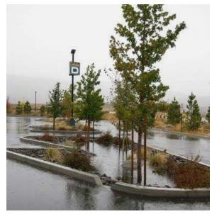
Fig. 33 Example of a curb cut for runoff collection
