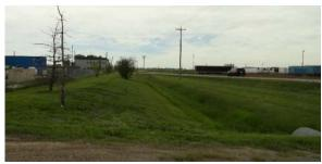
Fig. 29 Vegetated drainage swale
