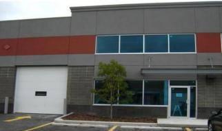
Fig. 20 Example of parapet wall
