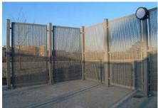
Fig. 38 Perforated metal panel fence
